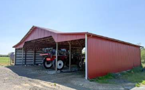
EQUIPMENT HAY SHED 70X60
