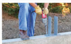
Sturdi-Wall™ Brackets Drill set for cured foundations
