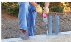
Sturdi-Wall™ Brackets Drill set for cured foundations
