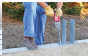
Sturdi-Wall™ Brackets Drill set for cured foundations
